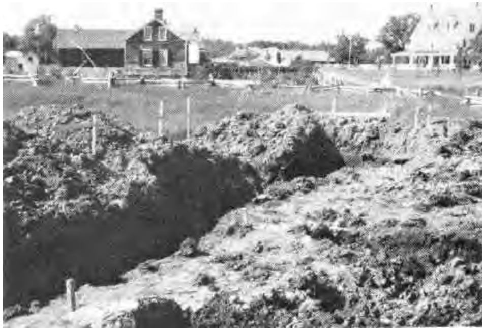
Figure 6. Trench for Victorian House foundation (photographed by Gordon DeAngelo).
