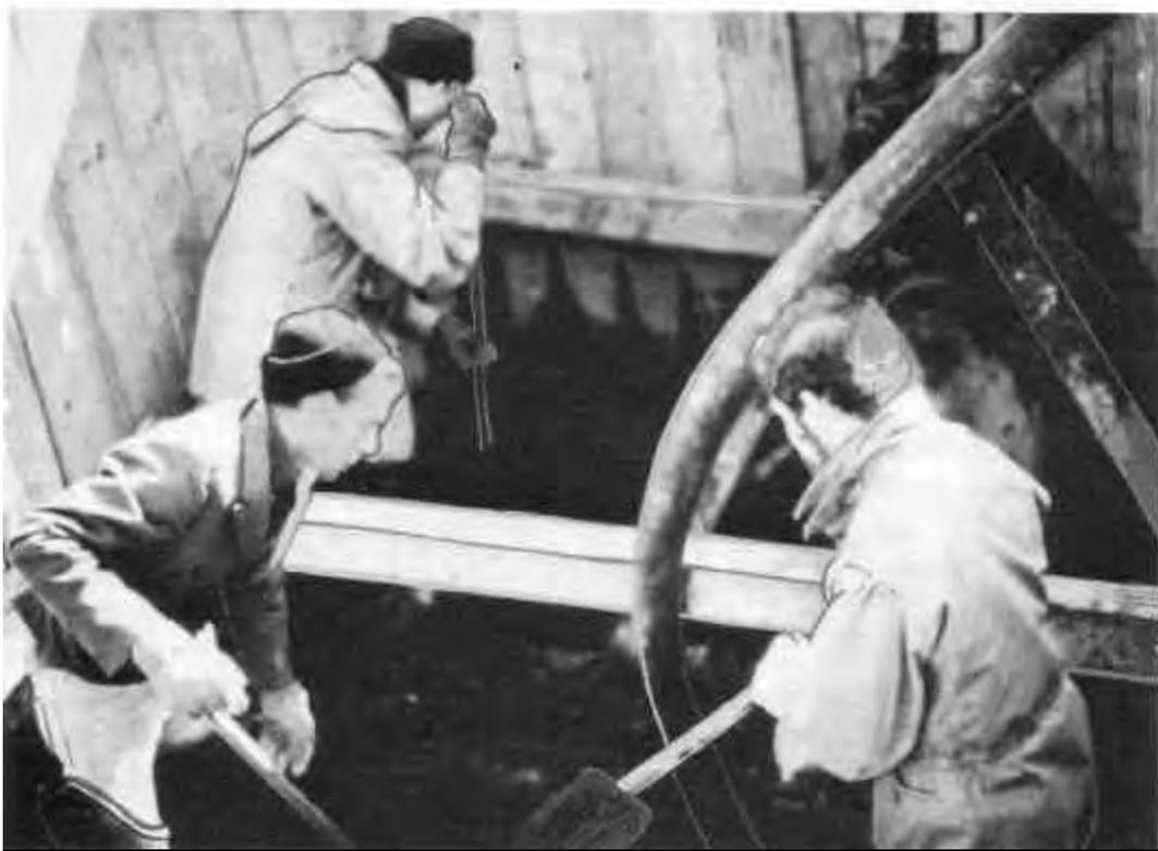
Plate I. Excavation Scene. Note sheathing, pump hose, and crane bucket.
