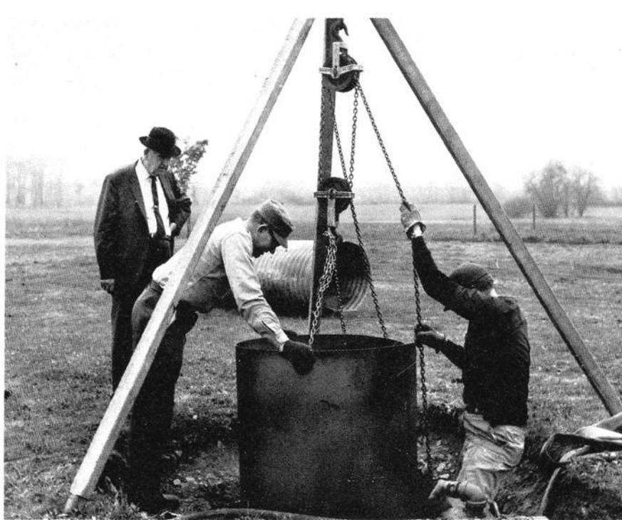
Fig. 1. Lowering the first section of pipe into the well.
