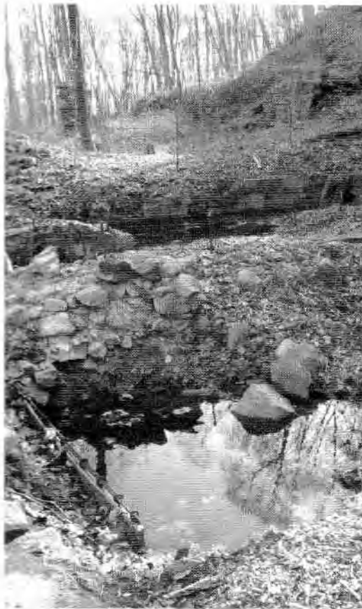
Figure 3. View south-by-southwest across the corrugated terrain of the Boring Mill foundations, from the plane and lathe area within an addition to the building. The wheel pit is in the foreground with the arched face of the tailrace temporarily covered by a sheet of plywood. The standing water in the background is the basement under the cannon boring beds. Photograph showing the corrugated terrain of the Boring Mill area at the West Point Foundry Site. Photo taken by Elizabeth Norris on April 9, 2007 and used by permission.
