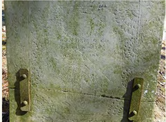
Figures 2 and 3. Examples of early gravestone repair using bolts and iron straps.
