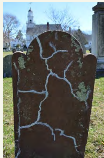
Figures 4 and 5. Examples of early gravestone repair using caulking and Portland cement.
