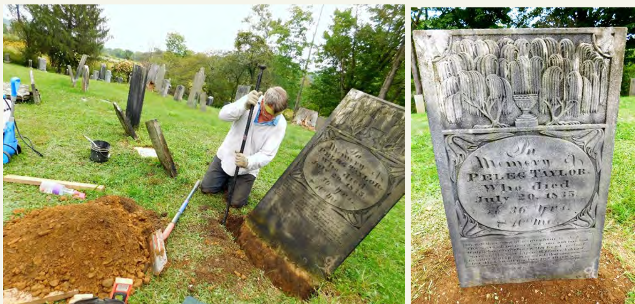
Figure 1. Before and after photographs shoeing gravestone straightening and cleaning.
