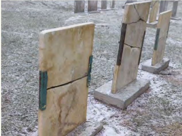
Figures 2 and 3. Examples of early gravestone repair using bolts and iron straps.
